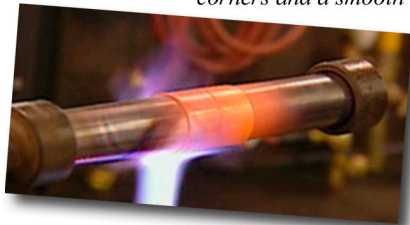
Brazers say a natural gas torch has better control and a more forgiving flame yet still provides plenty of heat
