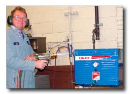
Torch Boosters are installed indoors with no special site preparation - just a simple connection to the utility natural gas pipe
