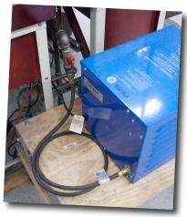
Torch Boosters come with a shut off valve and a flexible hose to connect to the utility gas pipeline.
